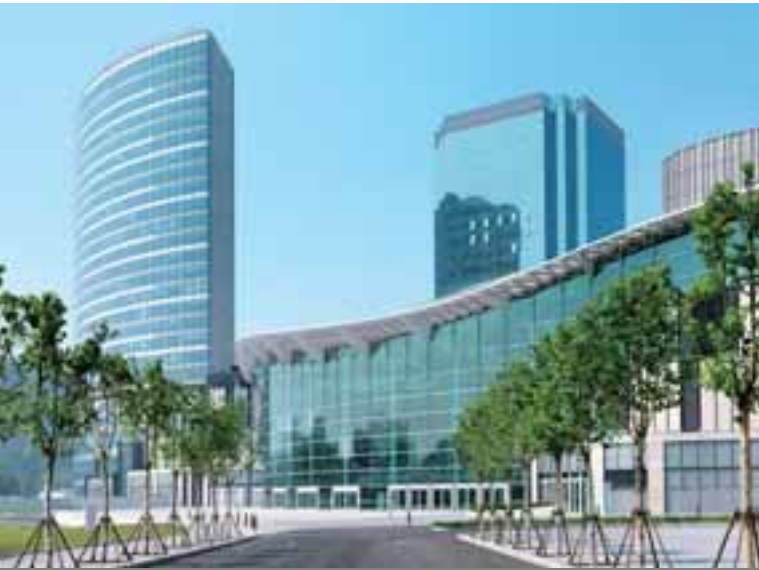
INDIGO, Swire Properties' new mixed-use development in Beijing, comprises a shopping mall, a Grade-A office tower – ONE INDIGO, and a lifestyle business hotel, EAST, Beijing.
