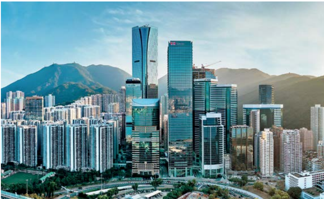
The redevelopment of Taikoo Place is an example of placemaking at its very best.
